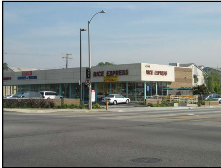
Exterior of Subject Property
